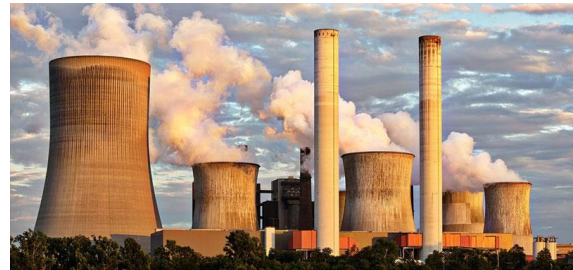
Figure.2. Thermal power plant
